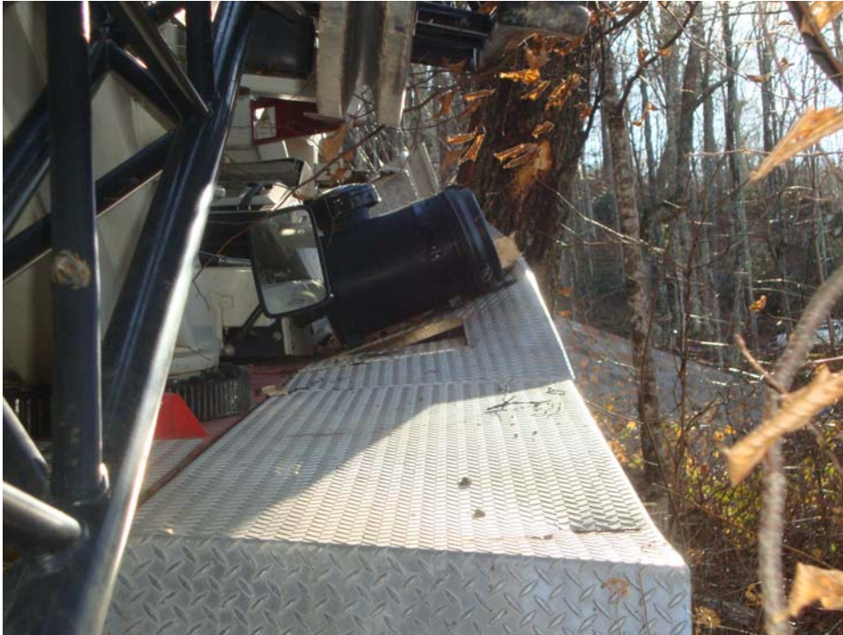
Photo #17: Additional view of platform decking.
