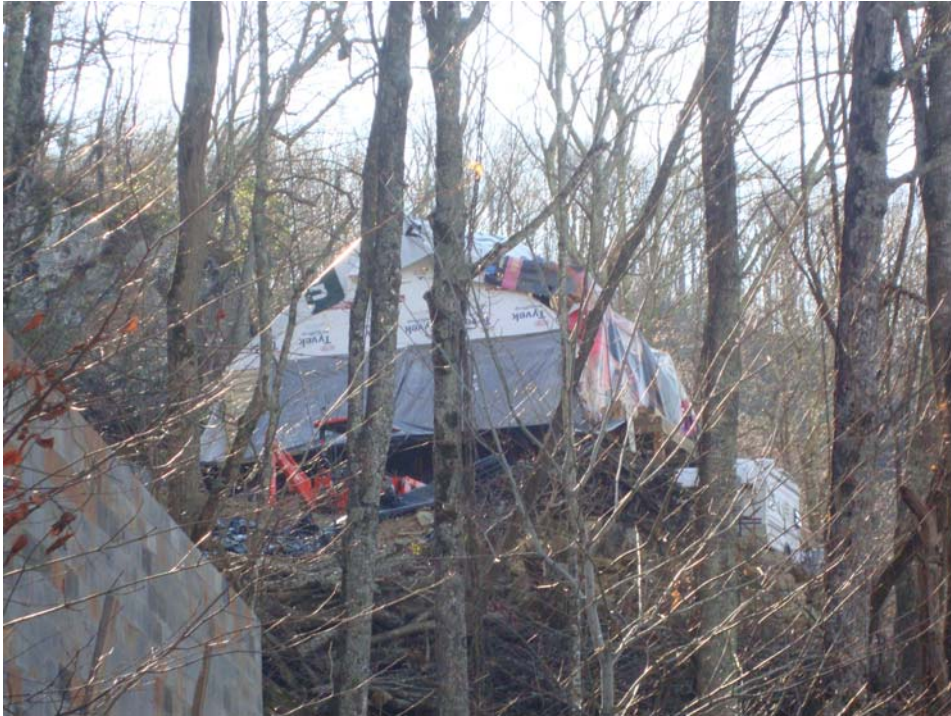
Photo #21: Insured's work included the truss erection for homeowner's new building on mountain site.
