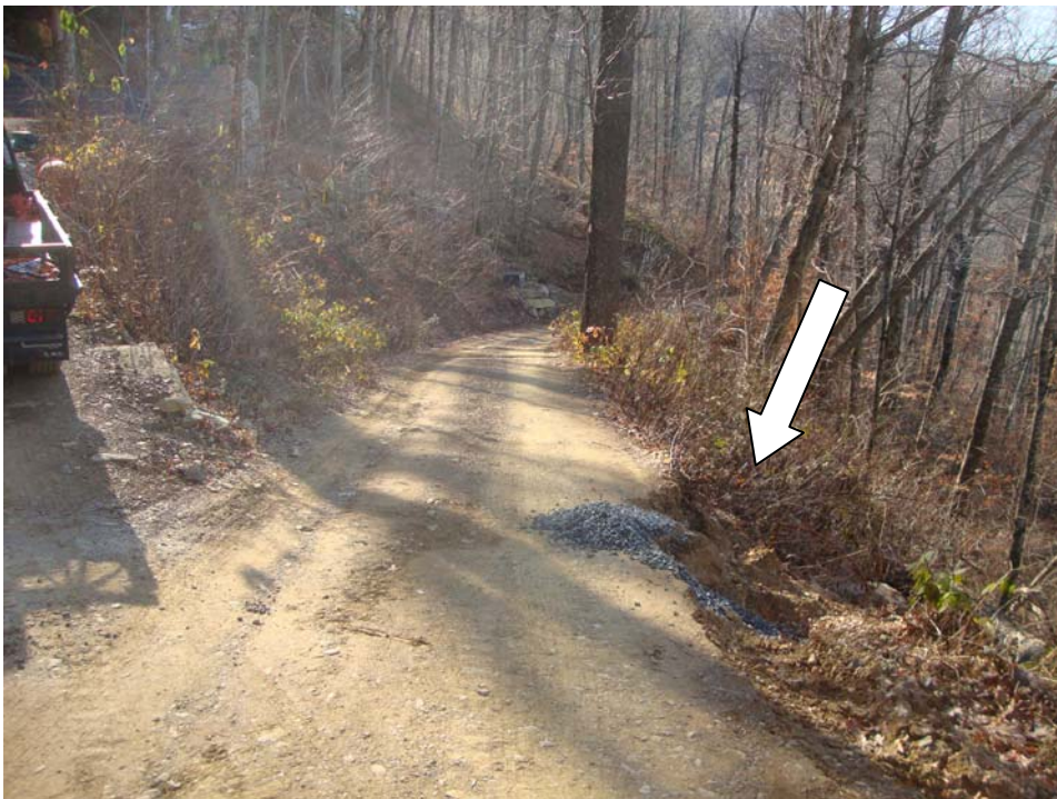
Photo #20: View of loss location. Insured was operating unit down driveway, hit soft spot and rolled over down mountain approx. 20'.
